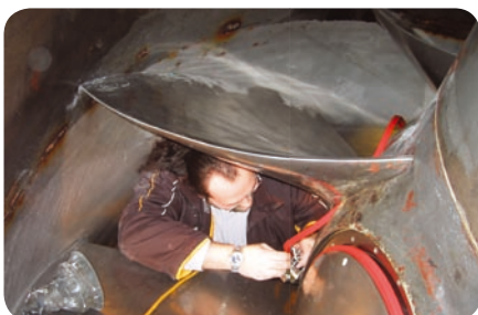
Step 1: Mounting of runner blade seals
