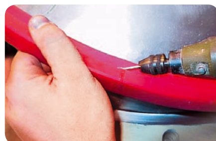
Step 5: Post-processing with special milling tool
